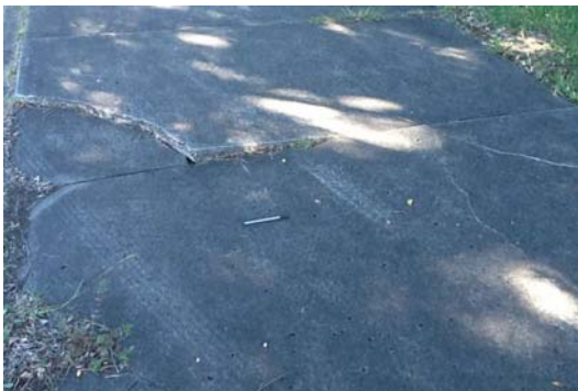
Burns Bay Road NB off-ramp (western side)
