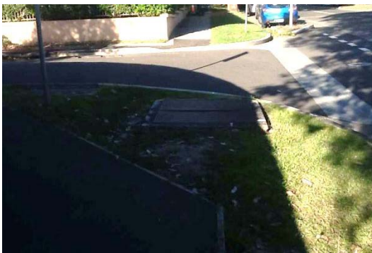
Gladesville Road (at Luke Street) not aligned
