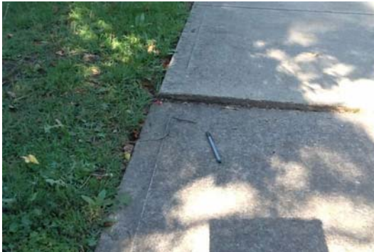
Matthew Street (western side)
