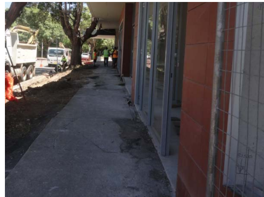
Photograph 2: Footpaths under transition adjoining construction sites
