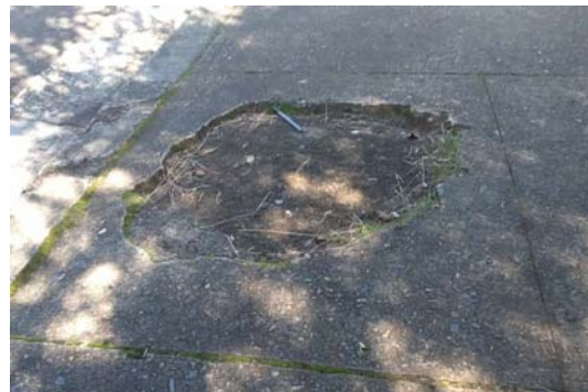
Reiby Road (western side)
