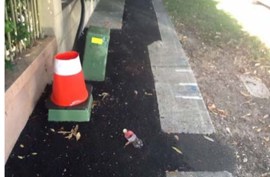
Gladesville Road (northern side)
