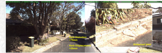
Tree Avenue, Hunter's Hill: Kerb Distortion and Displacement
