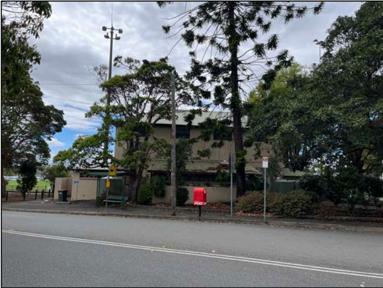
Figure 7 Pavilion Building – rear elevation as viewed from Park Road, looking east
