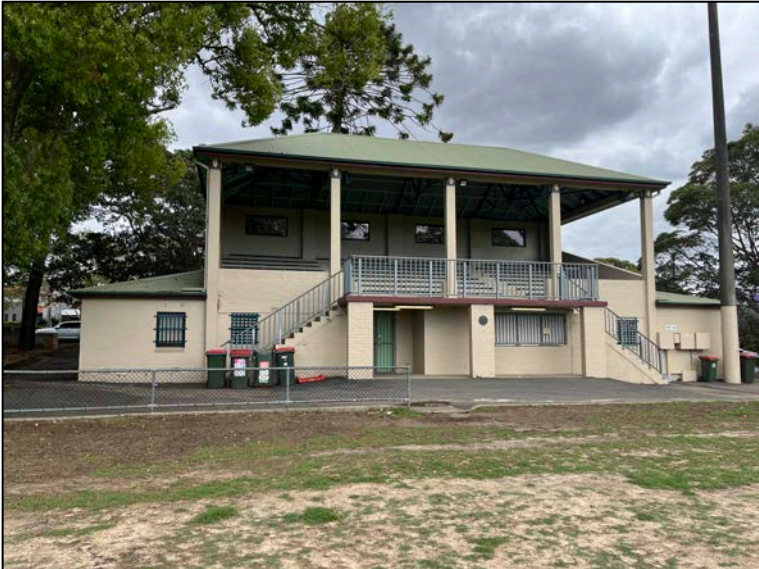
Figure 10 Boronia Park Pavilion – front elevation as viewed from the Park Cricket Oval
