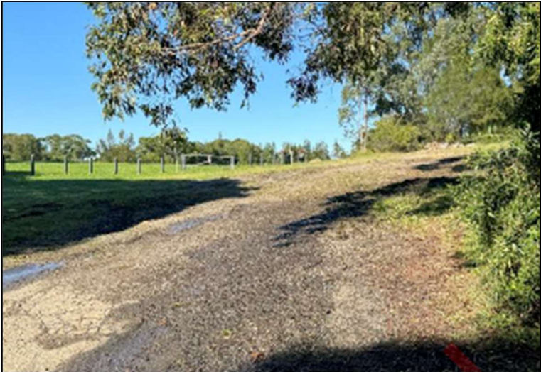
Figure 8 Existing access road looking south towards Oval 3
