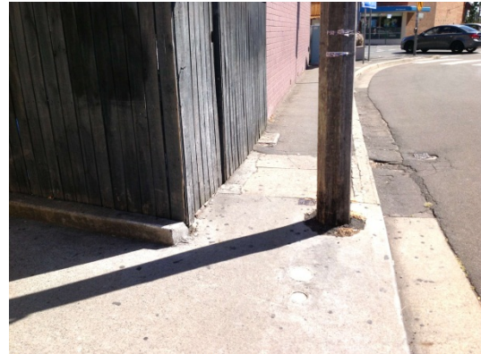
Photograph 11: Massey Street, between Massey Lane and Victoria Road (south side)
