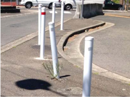
Photograph 8: Wharf Road/Meriton Street
