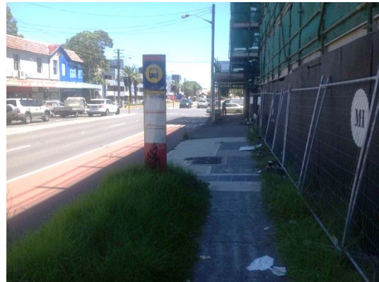
Photograph 19: Victoria Road, at southeast corner of intersection at Monash Road
