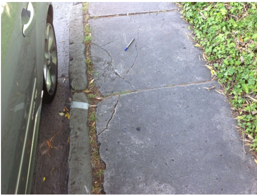
Photograph 6: Massey Street, between Massey Lane and Flagstaff Street (north side)
