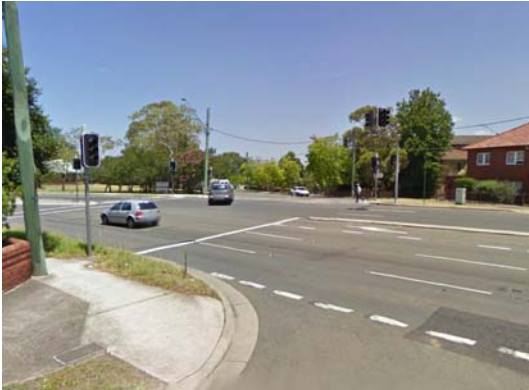
Photograph 27: Victoria Road, between Punt Road and Meriton Street
