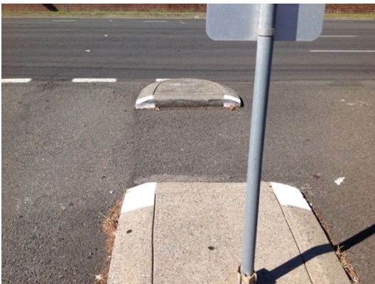
Photograph 25: Manning Road, north of Victoria Road intersection
