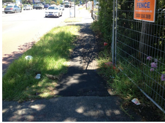
Photograph 5: Victoria Road between Monash Road and Tennyson
