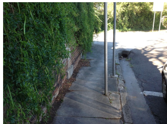
Photograph 13: Massey Street, between Massey Lane and Flagstaff Street (north side)
