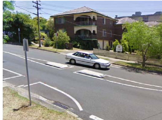
Photograph 24: Cowell Street, west of Flagstaff Street intersection
