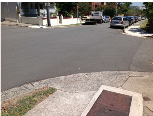
Photograph 14: Linsley Street, at south corner of intersection at Orr Street
