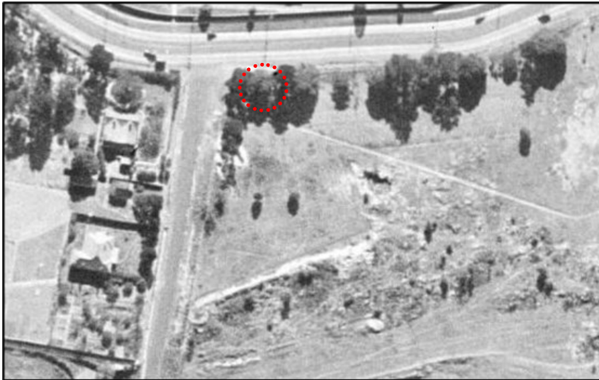
Aerial image 1943 Image Source: NSW Government Historical Imagery
